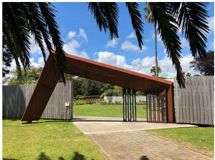
Figure 13: Homestead Garden Entrance – Functional Sculpture
